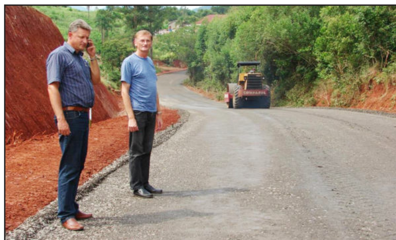
Hércio e Ariberto (e) conferem as obras
