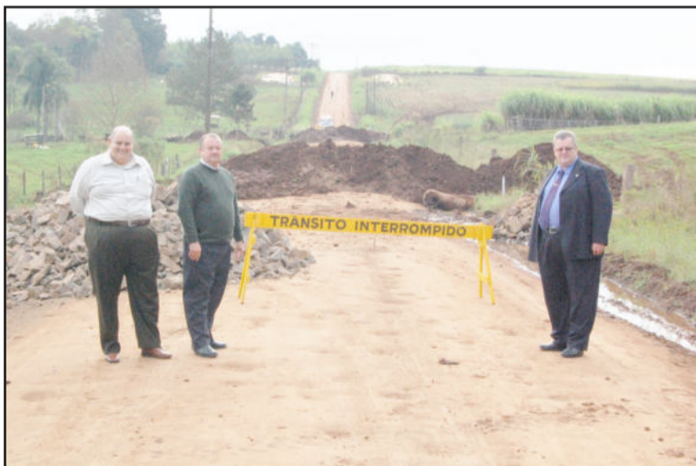
Cerne (e), Dickel e Althaus visitam as obras
